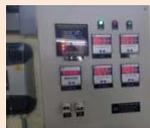
Department of Electrical Engineering sets up the system consists of One Horizontal Axis 3.8 KW @ 48V, Wind Turbine coupled induction Generator, 4 KW (500 W × 8) Solar Panels @ 48V. The Co-generated Energy is converted to DC and combined in a DC Bus. Which in turns run a Grid Tied true Sine Wave Inverter and Excess Energy after catering the Load of Two Labs is used to charge the Storage Battery rated at 48 Volt @ 400 AH.
